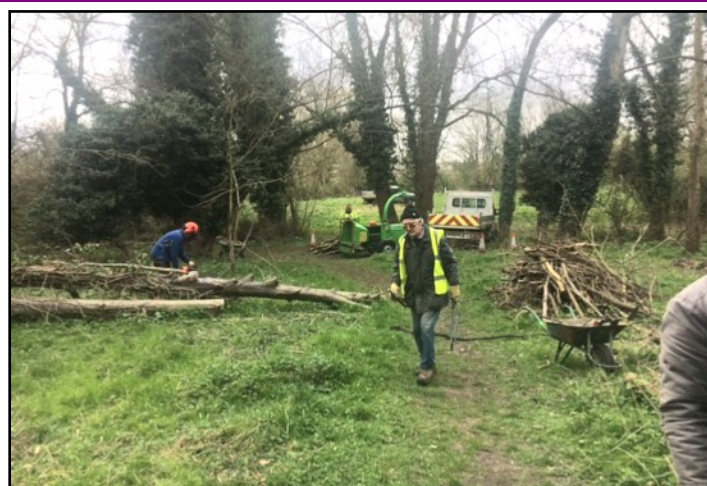
Clearing fallen timber close to the new nature area
