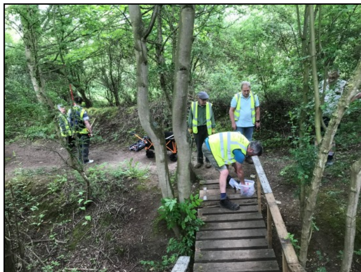
Repairing the footbridge at the Nature Reserve
