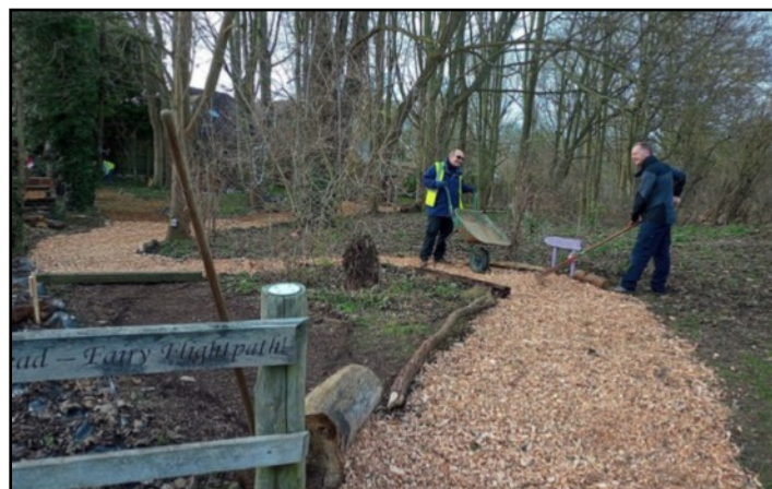
Resurfacing the Woodland Walk at the Mill
