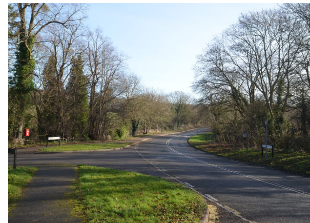
Figure 08: Northampton Road, a secondary road in the parish which leads from the A428 into the village.
