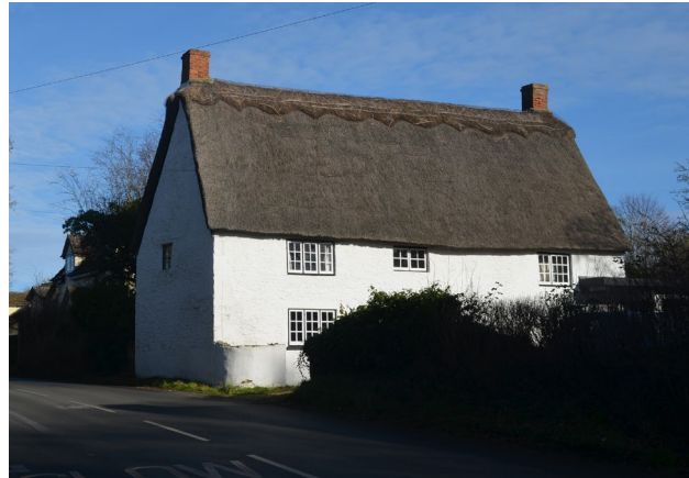
Figure 49: 17/18th century thatched house with colour-washed course limestone rubble and part roughcast over timber frame.
