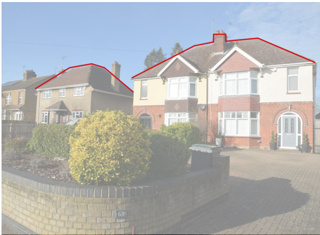
Figure 26: Hipped roof two storey houses on Molivers Lane.
