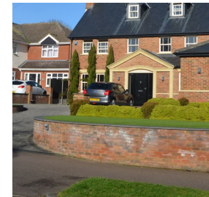
Red brick wall
