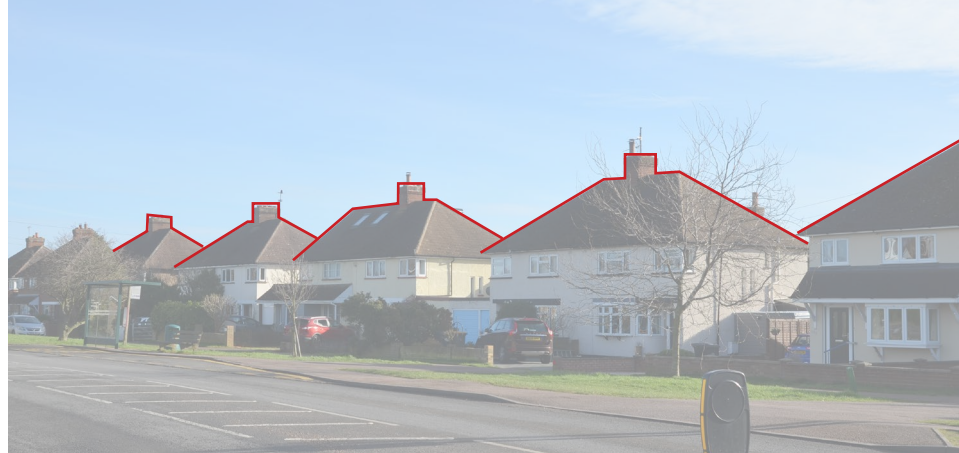
Figure 25: Hipped roofs of two storey houses along Stagsden Road.
