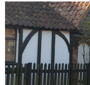
Exposed timber framing
