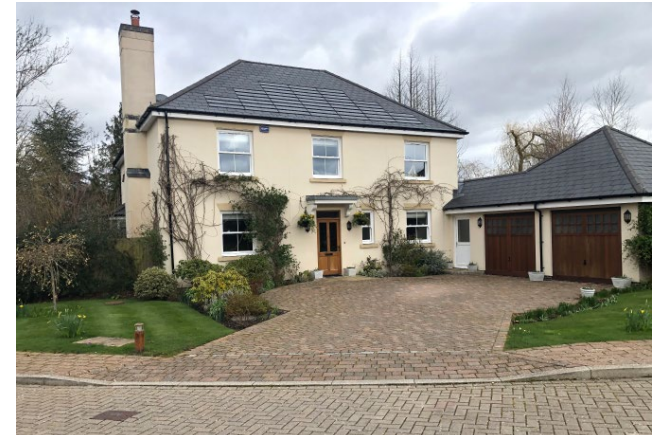
Figure 59: Use of shingle-like solar panels on a slate roof, with the design and colour of the solar panels matching those of the adjacent slate tiles.
