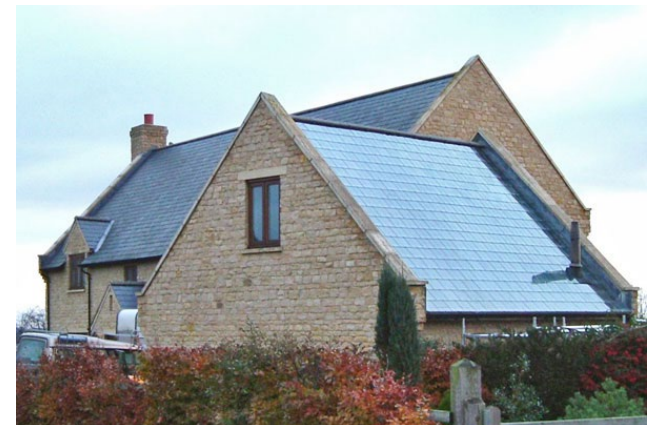
Figure 60: Positive example of implementing solar panels since the design stage.
