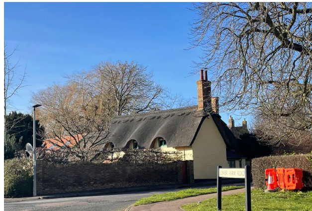
Figure 51: 18th century cottage, muted yellow colour washed roughcast over timber frame with a thatched roof and two yellow brick end chimney stacks.
